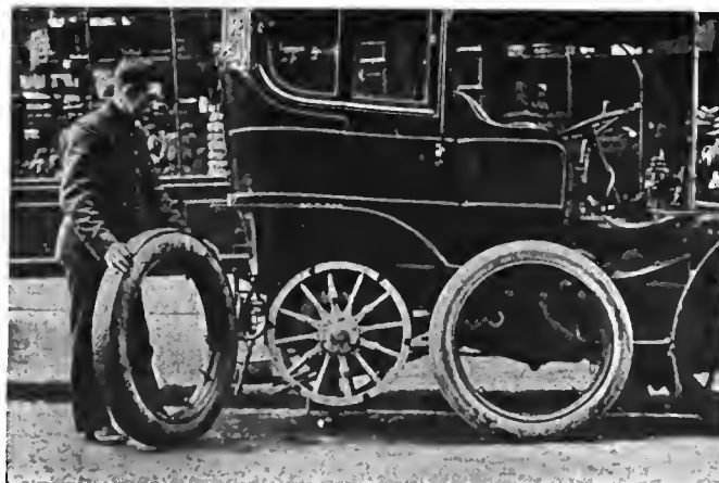
THE M. L. RIM WITH TIRE REMOVED.
